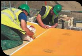
Temporary Floor Protection has developed a system called TecDura (pictured) that protects precast concrete staircases and high-quality finished concrete floors during construction phases. "[This anti-slip] mat is more robust and easier to use than traditional forms of protection such as corrugated plastic, bubble wrap and plywood to stop dirt, grit, grime and liquids from damaging finishes," says James Galloway, Managing Director, Temporary Floor Protection.
